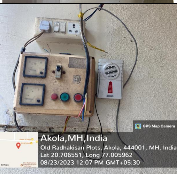
Sensor-based energy conservation: Water tank overflow alarm system installed at three places in college campus.
