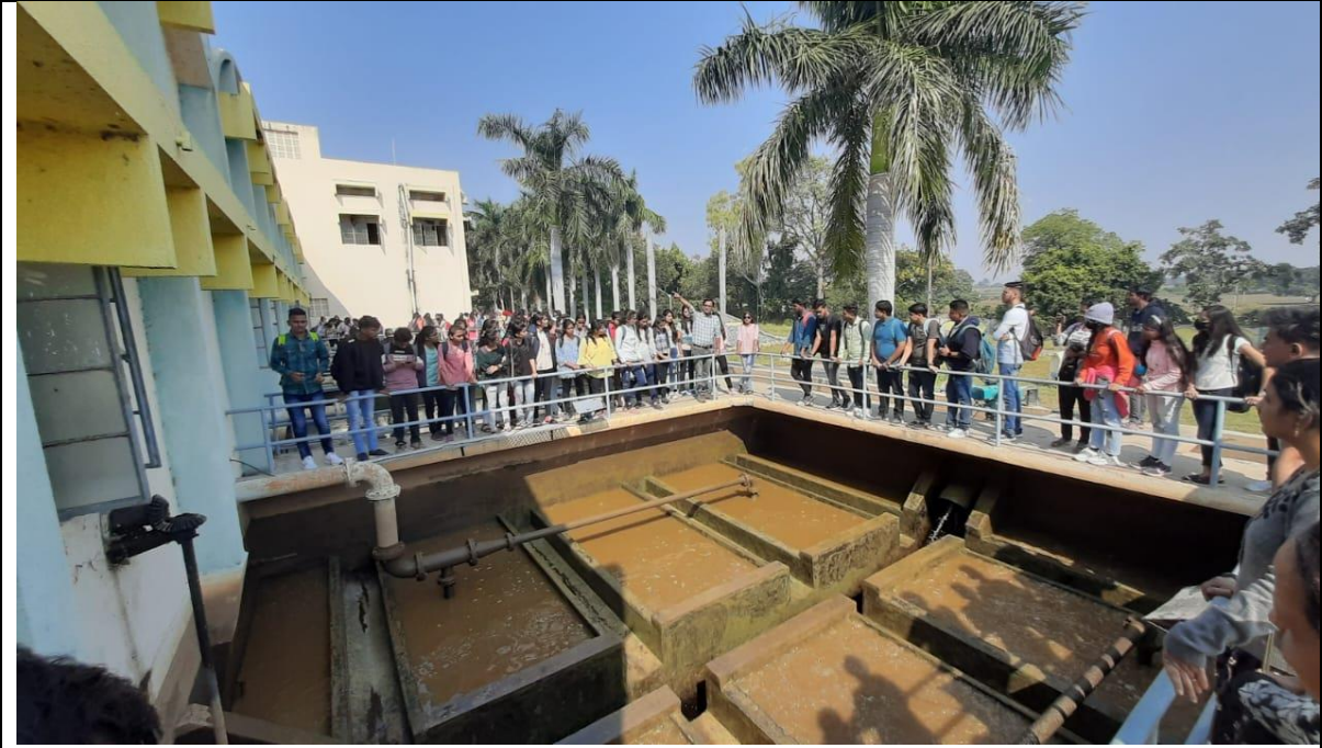
Rapid Sand Filter Beds During The Process Of Backwashing
