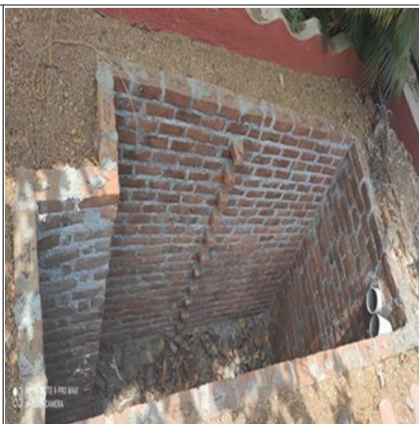
Waste water to soak pit through underground drainage from P.G. Laboratory of Chemistry.
