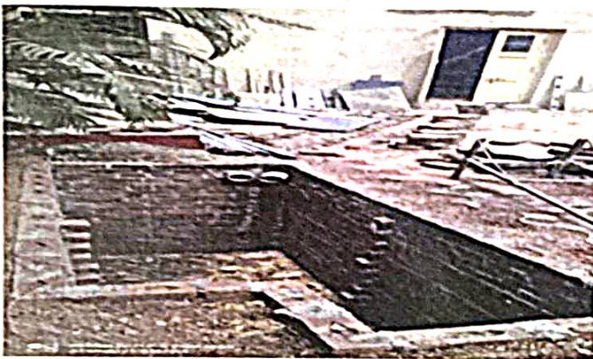
Waste water to soak pit through underground drainage from P.G. Laboratory of Chemistry.
