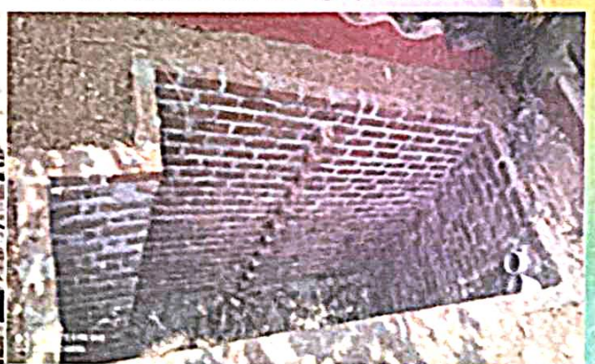
Waste water to soak pit through underground drainage from P.G. Laboratory of Chemistry.
