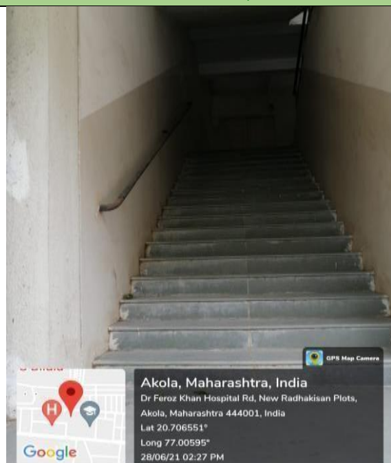
Ramps and Rails towards Library
