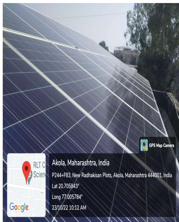
Solar panels of 18 kw and 12 kw on college main building
