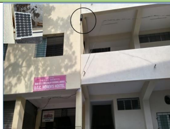
Solar based LED lights in campus
